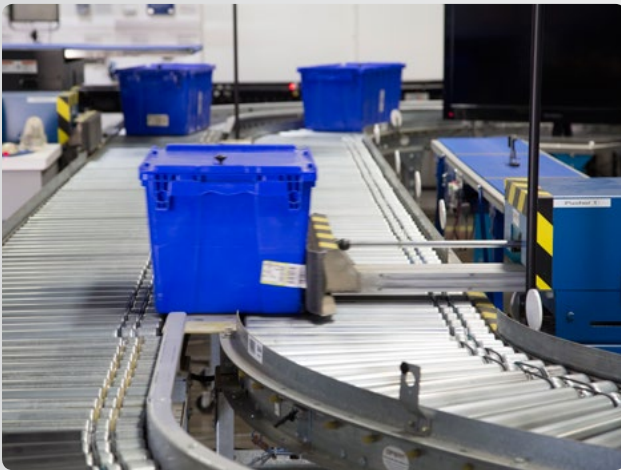
Gaps, safety hazard
